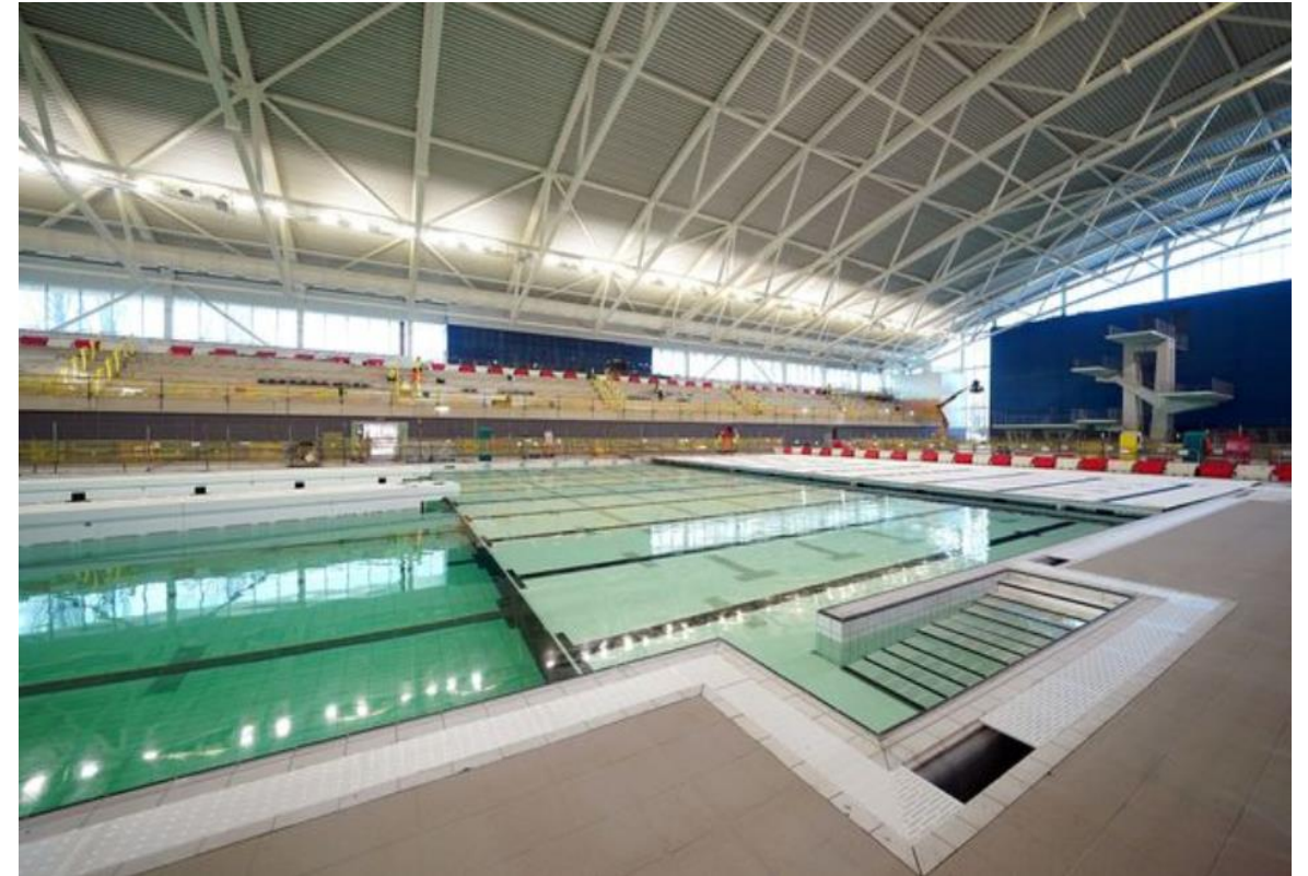
Main pool, diving pool and temporary 25m training pool with separate plant room. Temporary spa pool for the divers
